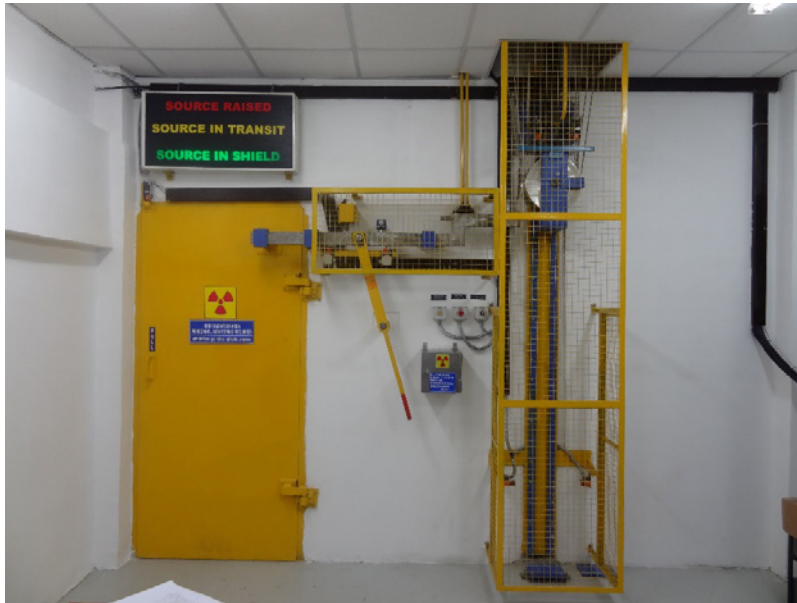
Figure 9: Access to the irradiator cell should be via a hardened security door fitted with opening detection sensors. Security can work hand in hand with safety, for example by interlocking a mechanical latch bar with the mechanism for lowering the source rack into a safe position as shown. The security of this mechanism, including encasement and tamper detection, should be considered. Illustration courtesy of Symec Engineers.
