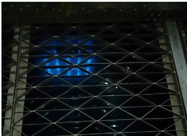
Figure 10: Access to the sources within the irradiator will be delayed by use of a pool cover. Various designs of solid covers or grills may be used and, in order to be effective, should be of hardened design, resistant to various tools, incorporate security fittings and not easily removeable by multiple attackers. Illustration courtesy of Symec Engineers.
