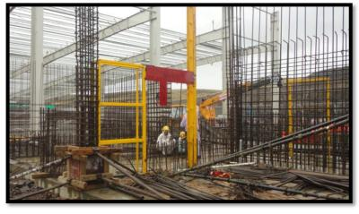
To operate in continuous mode, a maze is necessary to prevent radiation from exiting.
