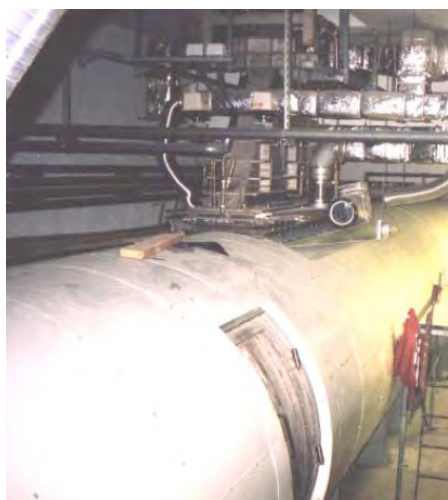
Figure 113. Flue Gas Irradiation Chamber with EB Unit
