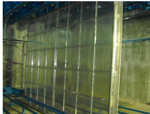
Figure 8: Source rack shroud (Courtesy of SQHL Radiation Engineering Technology Co., Ltd)
